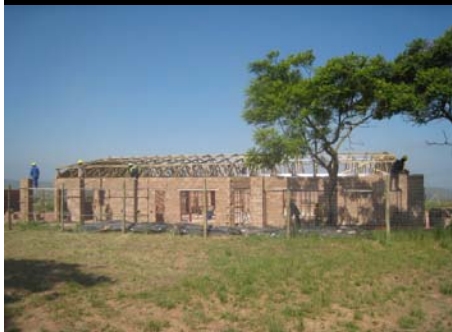
Mophela Clinic under construction in South Africa
