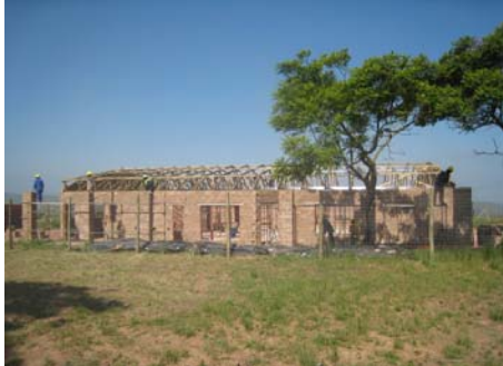
Mophela Clinic under construction in South Africa
